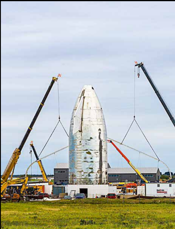
After Mk1's bulkhead shot into the sky during a pressure test in November, SpaceX began dismantling it, while speeding up production of its next prototype.
