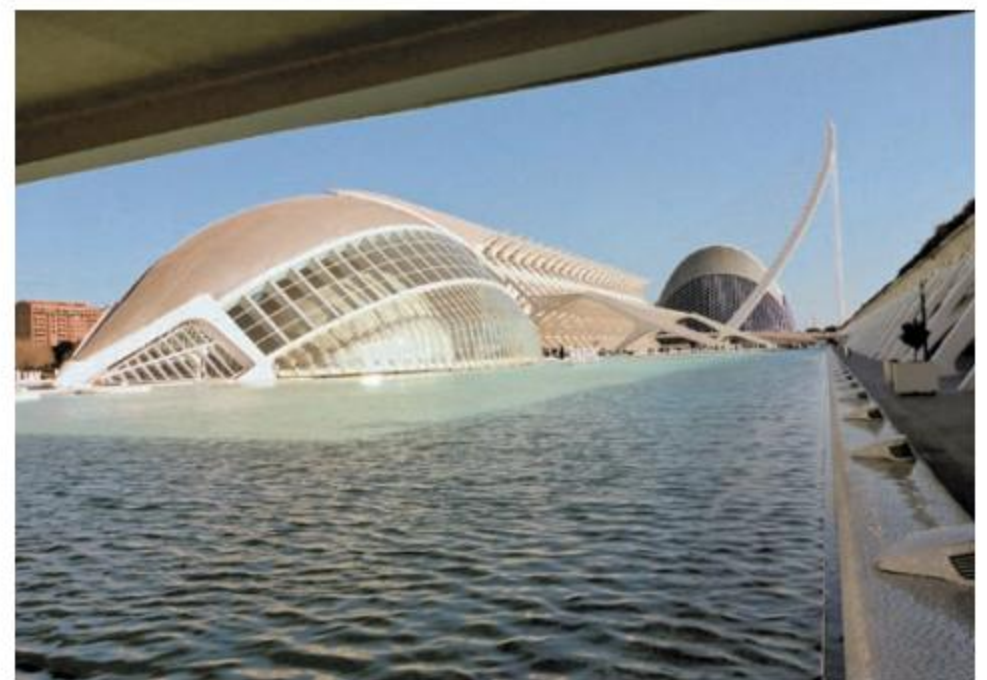
City of Arts and Science Complex in Valencia, Spain
