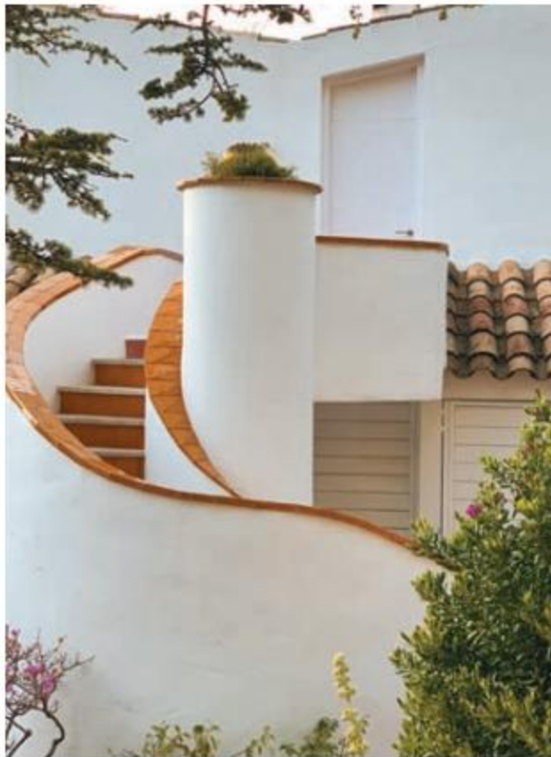
Outdoor application of tile, Spain
