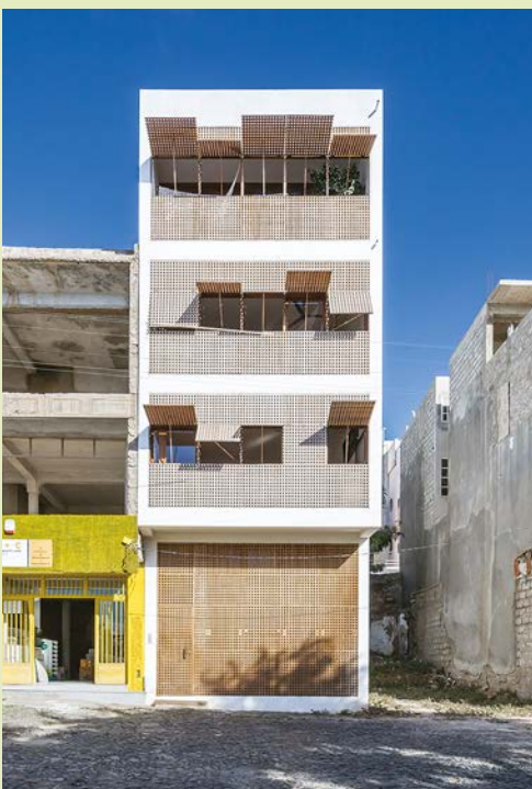
Terra Lodge's generous patios (above) offer unparalleled vistas of the surrounding landscape. The "pixellated" wood facade was informed by the architects' interest in the mashrabiya s — Islamic screens native to North Africa — they first explored in the 2009 residence Appartamenti Paz (left).
