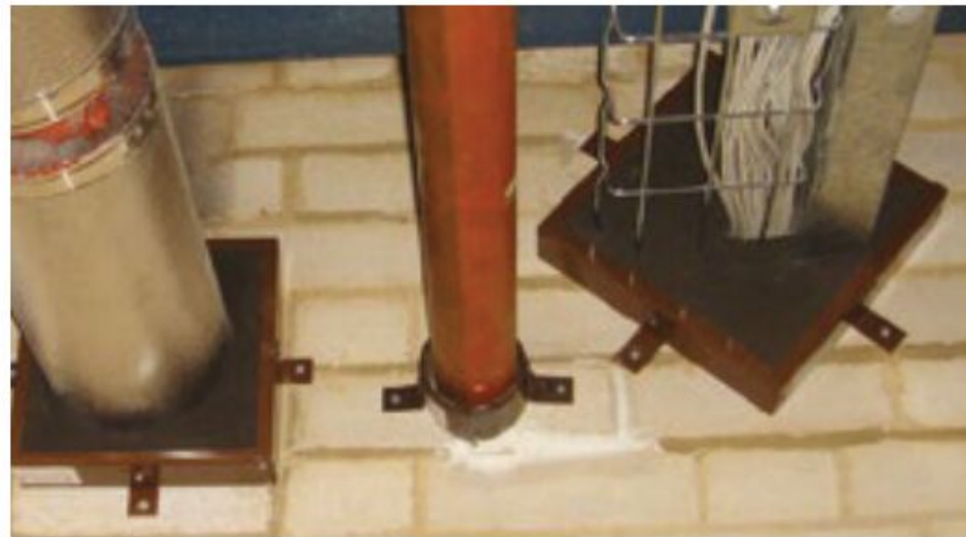
SERVICES THROUGH COLLARS & MULTI PURPOSE BOXES
