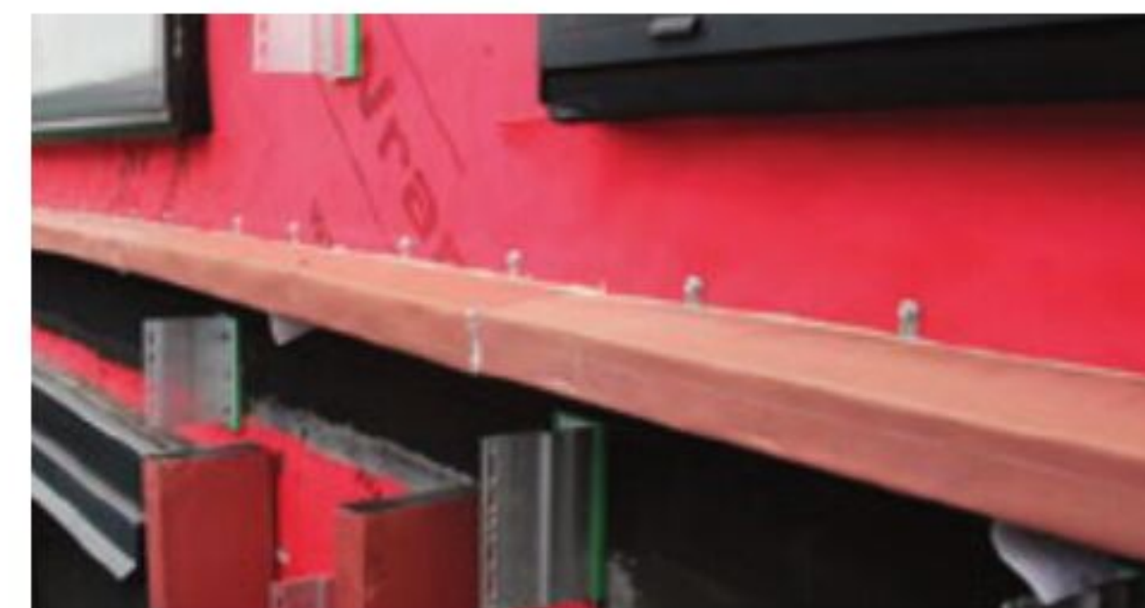
RSM - CAVITY BARRIER FOR RAINSCREEN FACADE SYSTEMS
