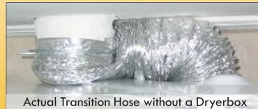
Actual Transition Hose without a Dryerbox
