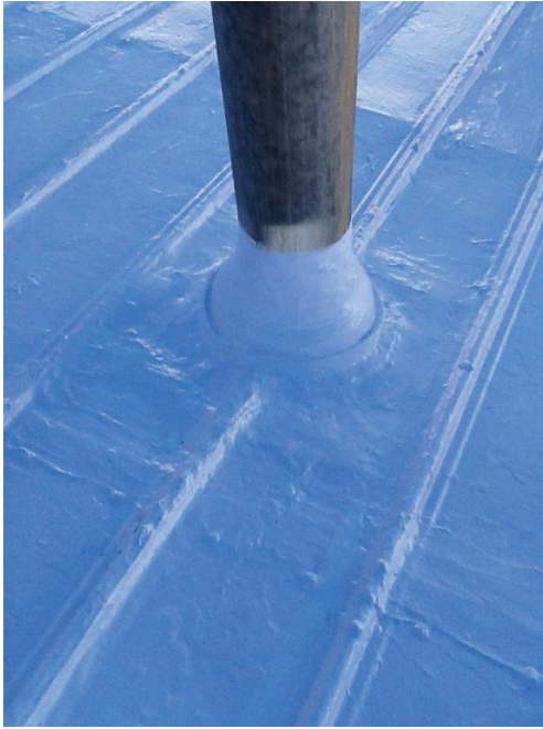
If there are multiple penetrations in a roof a fluid-applied coating can be a great choice, as the product is easily applied around the penetrations to form a seamless monolithic waterproofing barrier. Photo courtesy of Neogard, a part of the Hempel group
