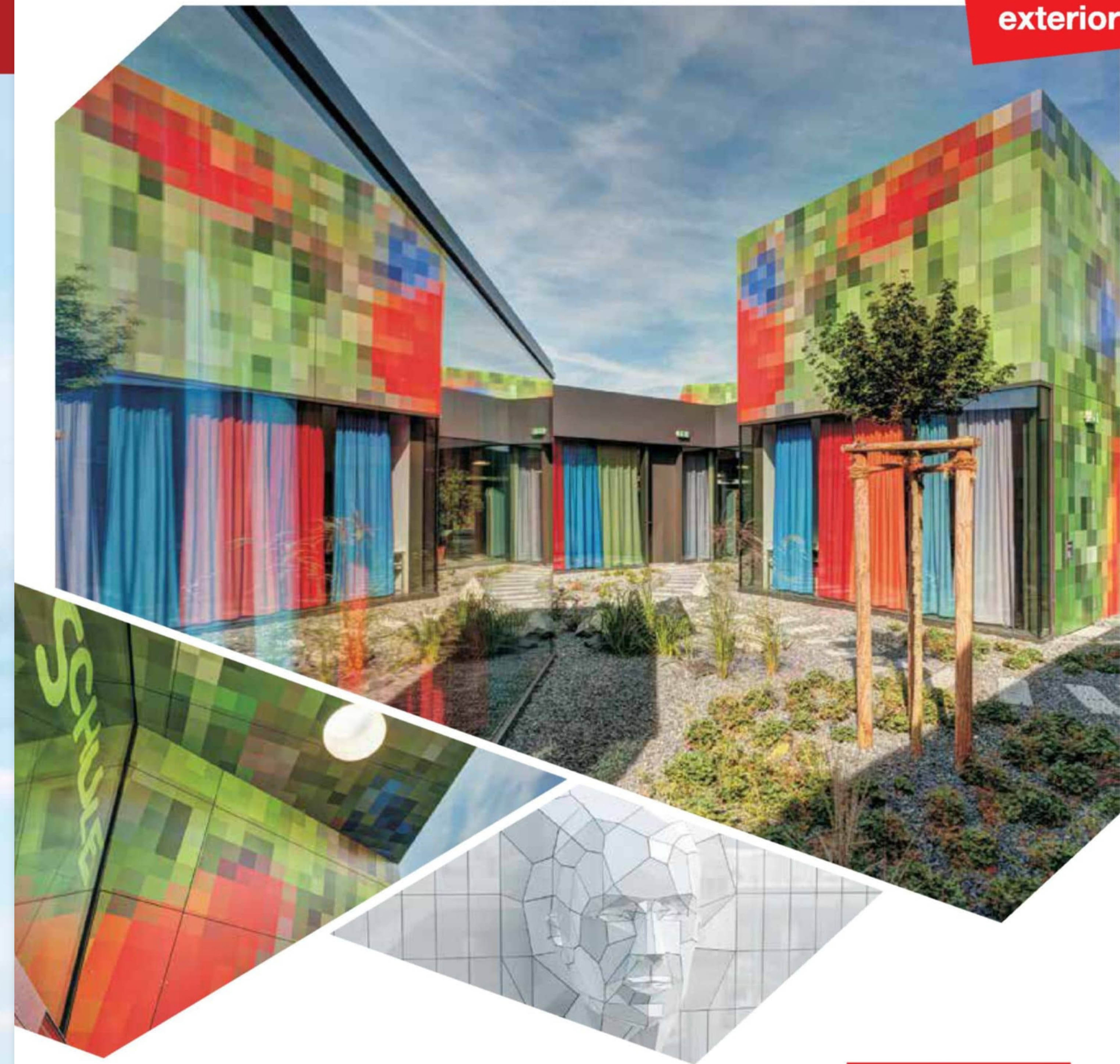
Primary school Sassenburg Westerbeck, Photo credit: thyssenkrupp Plastics GmbH, Architect: Augustin und Frank Architekten
