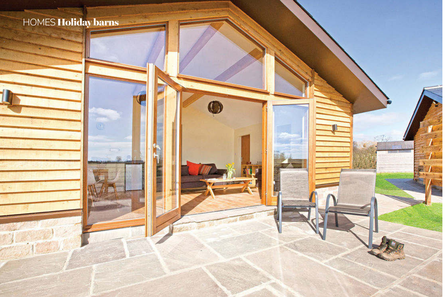
The barns were built using SIPs clad in green oak to blend with the surrounding countryside.
