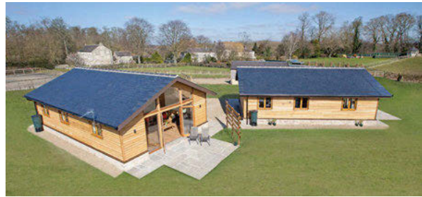
The barns were built using SIPs clad in green oak to blend with the surrounding countryside.
