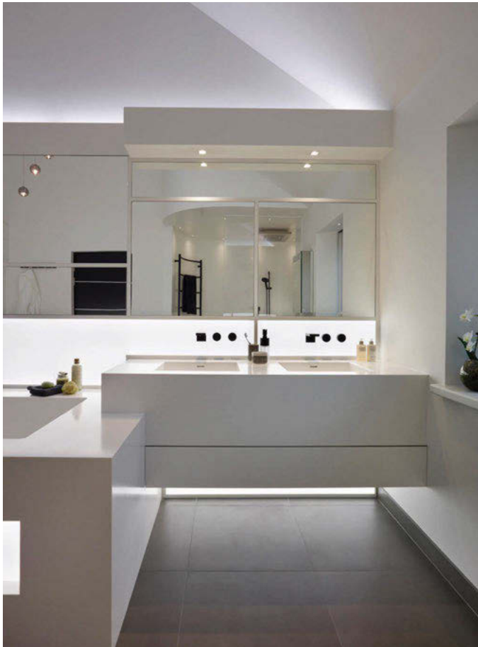
This entire bathroom was clad in Corian, attached to a timber-and-ply studwork frame and chemically bonded to eliminate joints. LED sheet lighting was placed behind thinner panels, which glow when illuminated.
