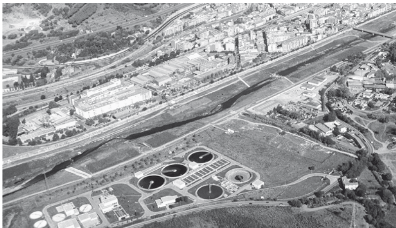
Figure 6.8. Sewage treatment facility by a river carrying considerable sewage wastewater. Large dark circles are secondary treatment tanks mainly for oxygenating wastewater to reduce organic matter with aerobic bacteria. Upriver the population far outstrips sewage treatment capacity. Small vegetable-garden plots in floodplain; sometimes midge populations (chironomids) in rivers are pests. During wet periods stormwater may fill or overflow the channelized-river concrete banks, sometimes causing huge floods. Note small access roads used by infrastructure maintenance vehicles and local residents. Besos River, Barcelona. R. Forman photo courtesy of Mark Montlleo.
