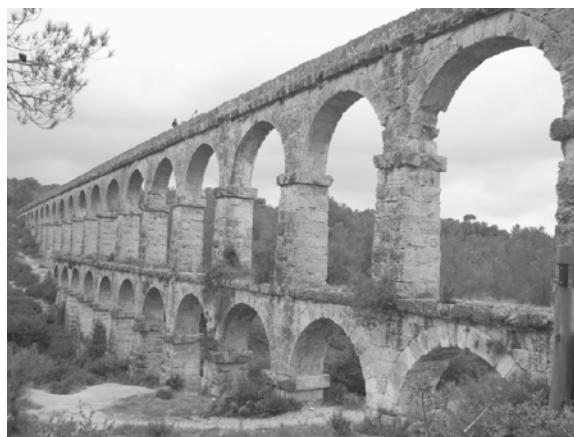
Figure 6.5. Aqueduct to carry clean water a few kilometers from a source to a Roman city. For the intermittent channel at bottom, water rushes over sand in wet periods, and slowly flows beneath the surface in dry periods. Built by Augustus Caesar ca. 25 BC; cut stones fit together without mortar. Tarragona, Spain. R. Forman photo.
