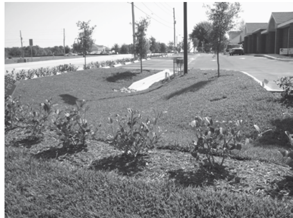
Figure 6.11. Small stormwater detention basin where runoff from roofs and parking lot accumulates. City of Lake Placid, Florida. R. Forman photo.
