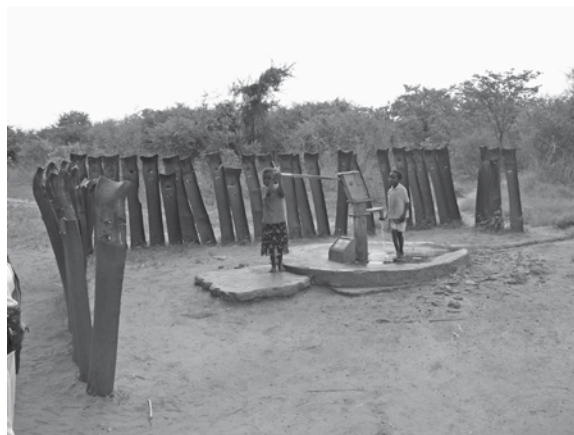
Figure 6.2. Community water supply pumped from groundwater. Steel pillars reduce problems with elephants that also wish to use the water. Peri-urban area of Livingston, Zambia. R. Forman photo.
