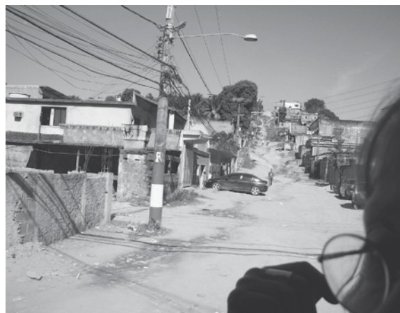
Figure 4.10. Erosion and line of wet soil in road of informal squatter settlement. Soil erosion due to both water and wind. The wet soil line during a dry period usually indicates community drainage of sewage wastewater. Favela on west edge of Rio de Janeiro. R. Forman photo.
