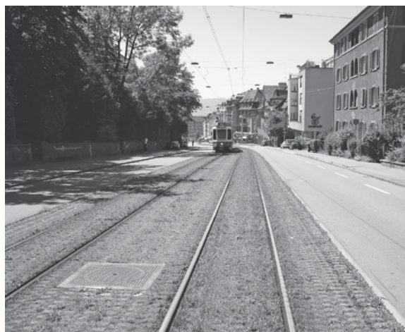
Figure 6.7. Electric-trolley public transit and manhole access to pipe system under street. Grass- and-block-covered surface to increase water infiltration and reduce heat buildup. Zurich, Switzerland. R. Forman photo.
