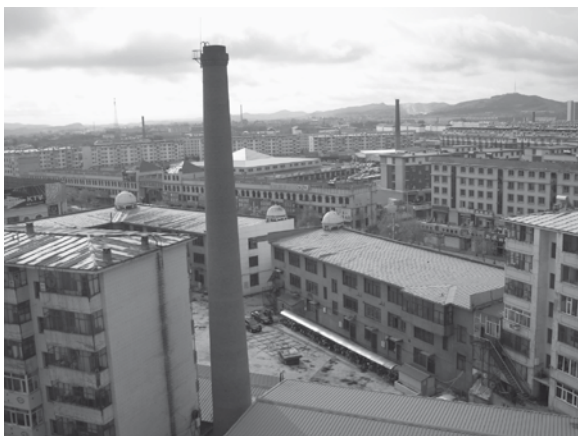
Figure 6.3. Smokestacks indicating power facilities heating water that is piped underground to buildings. White roof in center reflects considerable solar radiation (high albedo). City in Jilin Province, China. R. Forman photo.
