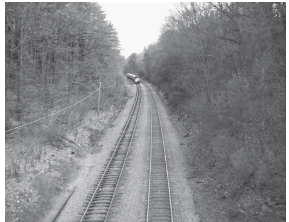
Figure 10.1. Commuter train, railway, and gravel bed with essentially no plants. Railway bank (left) with soil erosion mainly related to vegetation cutting under powerline; (right) with little managed trees and shrubs. Outer suburb of Boston, near Henry David Thoreau’s 1840s cabin (and periodic walking route home for dinner). R. Forman photo.
