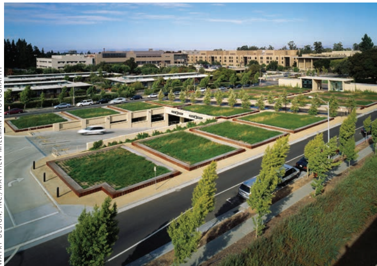
Landscaping on top of the 1,033-stall underground Stanford University Medical Center Parking Structure 4 reduces the heat island effect and helps to manage stormwater.
