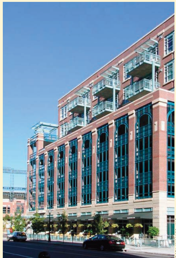
In order to integrate parking, retail space, and residences in the 1890 Wynkoop Building in Denver, a cast-in-place post-tensioned structural system was used.
