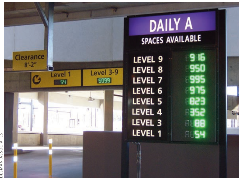
At Baltimore/Washington International Thurgood Marshall Airport, wayfinding is assisted by a space-counting system that lets drivers know how many spaces are available on each level.
