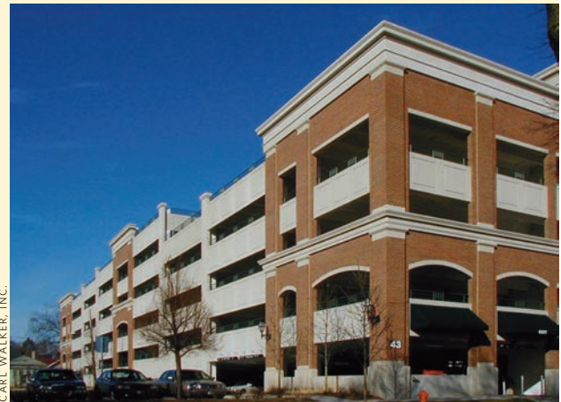
The VanBuren Street parking structure in Naperville, Illinois, was constructed with precast concrete.
