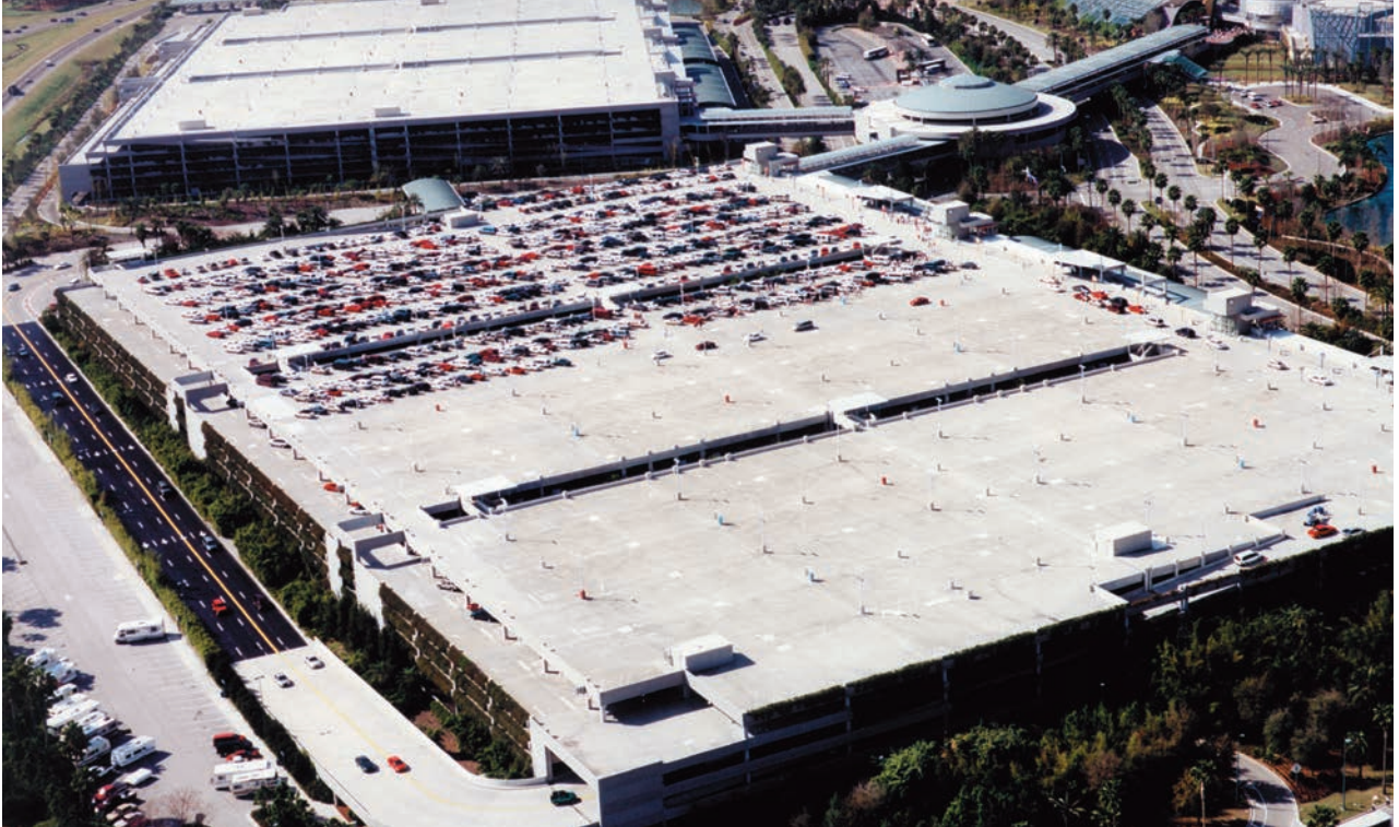
In Orlando, Florida, the north and south parking structures at Universal Studios have space for 19,423 vehicles.
