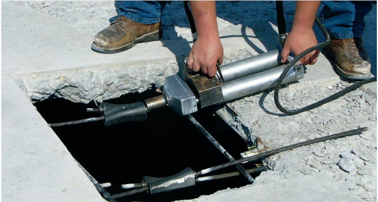
Replacement of broken tendons in a post-tensioned slab.
