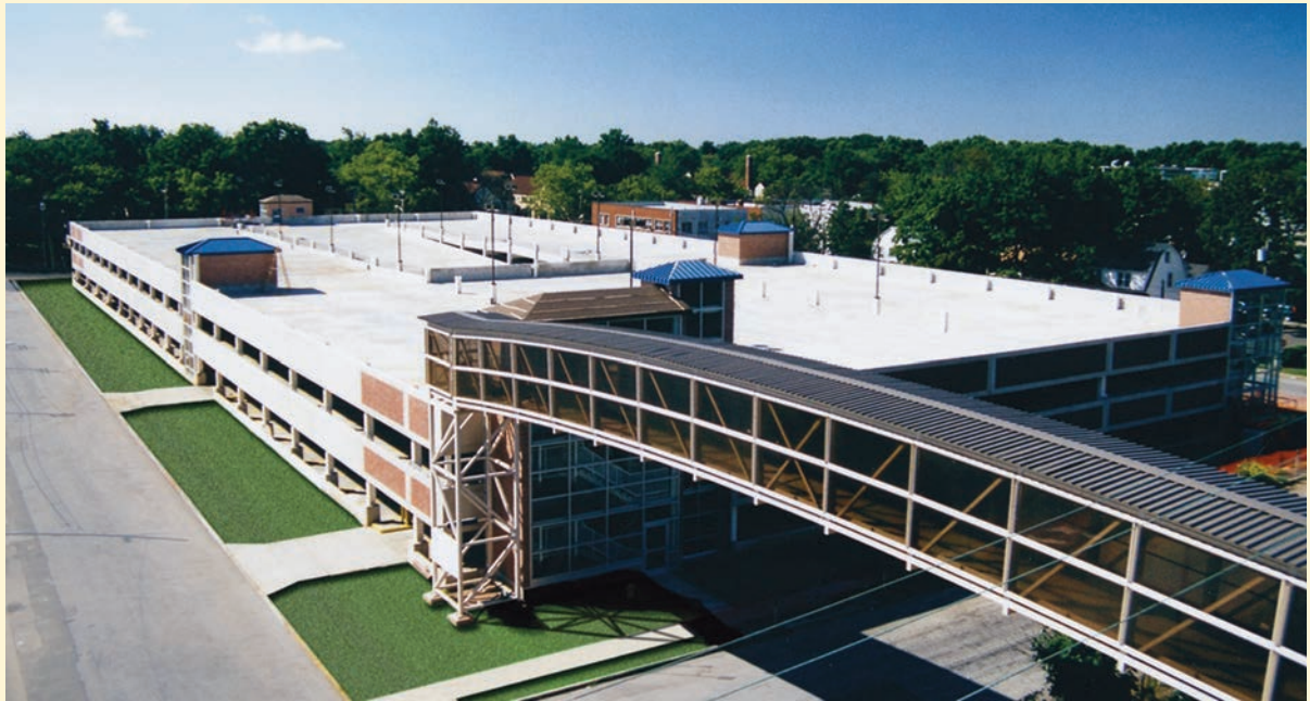
The Winthrop-University Hospital employee parking facility in Mineola, New York, has a steel-framed structure with a post-tensioned floor slab.
