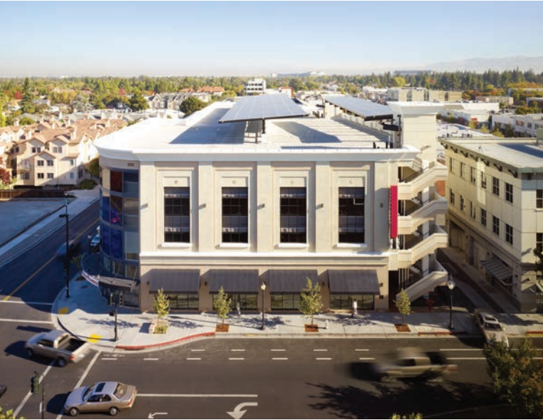
With a rooftop photovoltaic system that powers lights and elevators, the City of Mountain View Parking Structure comprises four stories of parking above 16,200 square feet (1,505 square meters) of streetfront retail space.
