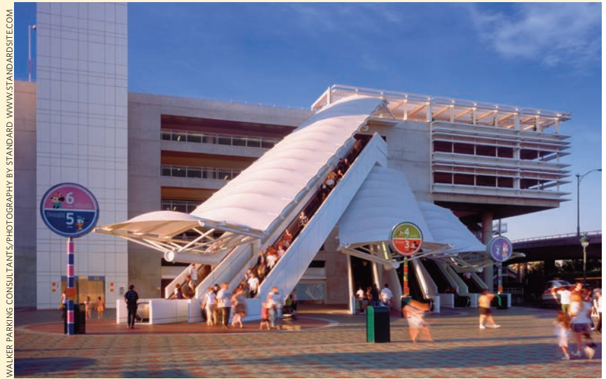
The Themed Entertainment Parking Building in Anaheim, California.
