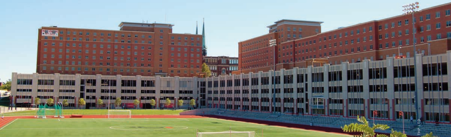
Bordering two sides of a running track and athletic field, the Calhoun Street Parking Garage in Cincinnati, Ohio, is a four-level, cast-in-place building with space for 1,000 vehicles.
