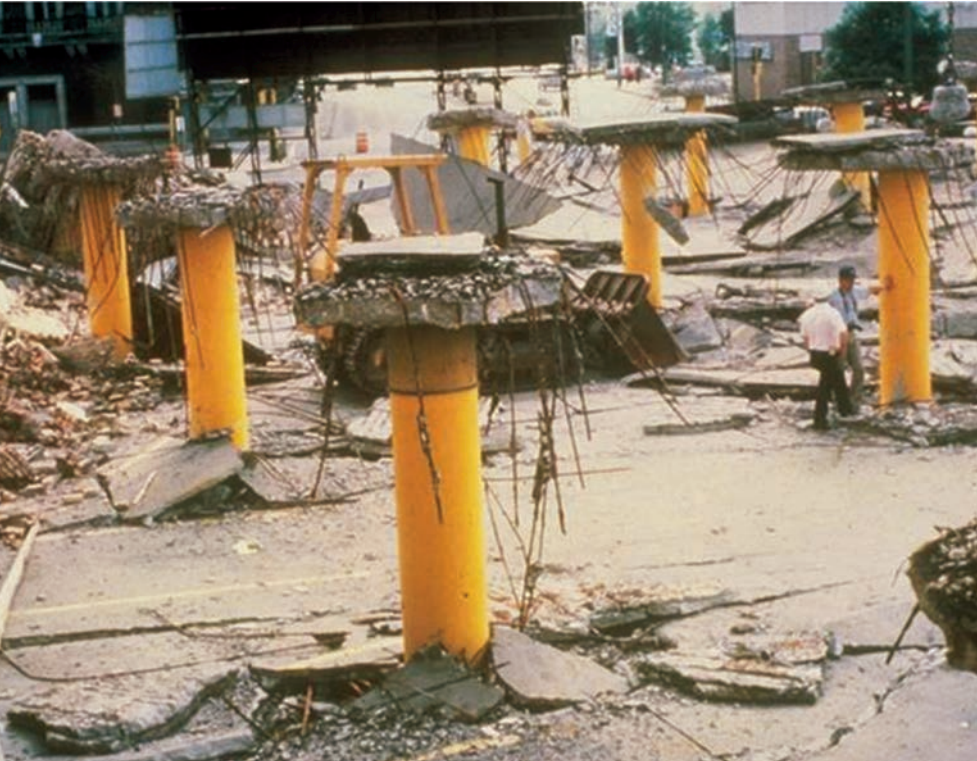
The worst-case scenario for a severely deteriorated garage is a collapse.
