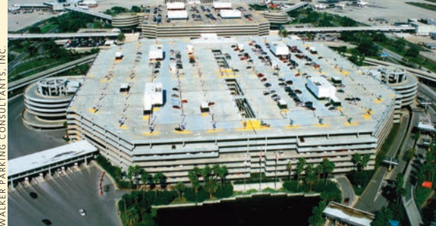
Cast-in-place post-tensioned concrete was used in the construction of the parking structure at Tampa International Airport in Tampa, Florida.
