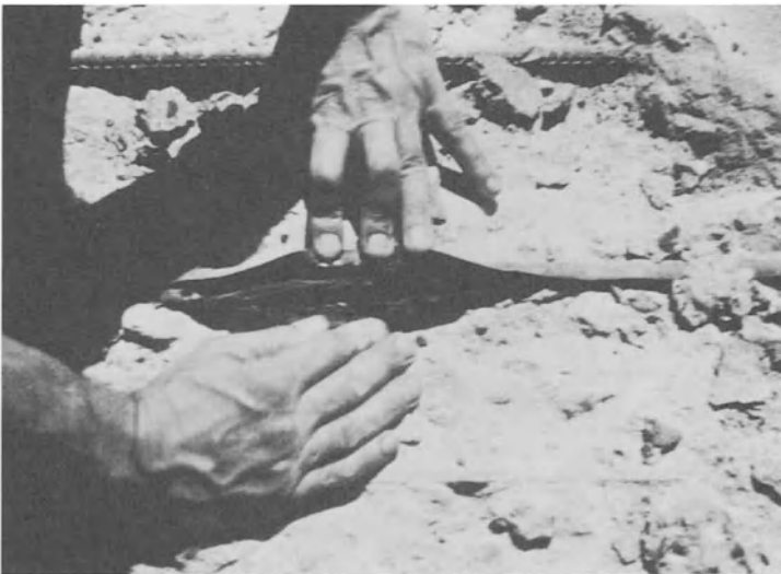
Figure 19-24: Strand with grease and push-through sheathing.
