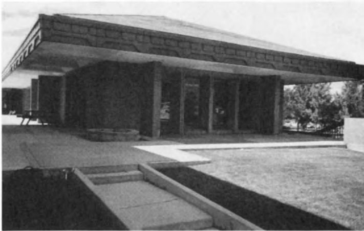
Figure 13-1: (a) Underground-parking facility with park and roadway. (b) Plaza deck with pedestrian walkway, landscaping, and building.
