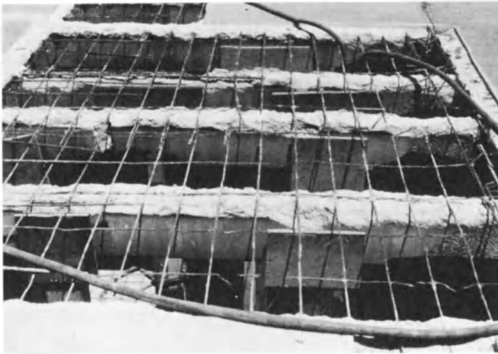
Figure 20-12: Full-depth slab removal (pan-joist system).
