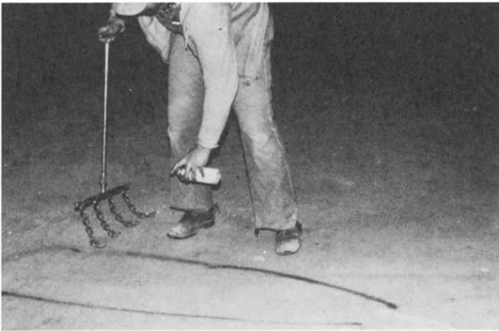
Figure 19-44: Chain drag delamination survey.
