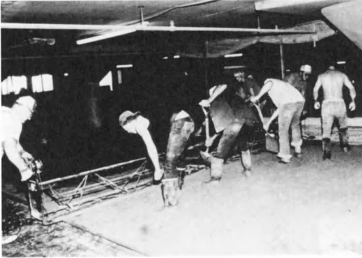
Figure 20-11: (b) Concrete overlay placement with vibratory screed.
