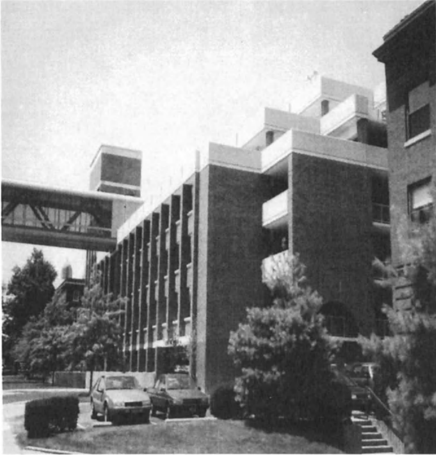
Figure 14-15: Barnes Jewish Hospital Parking facility, St. Louis, Missouri
