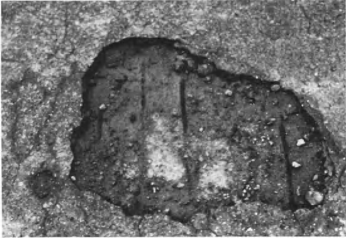
Figure 19-5: Concrete spall.
