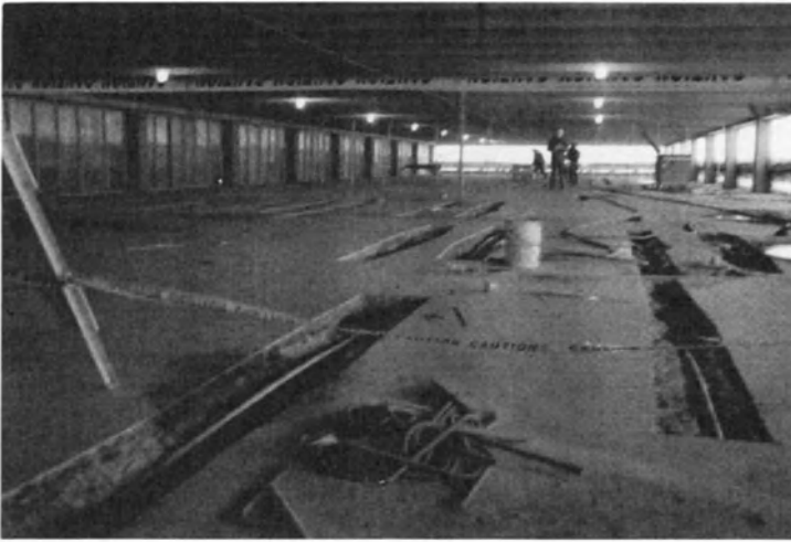
Figure 20-27: Trench method for tendon replacement.
