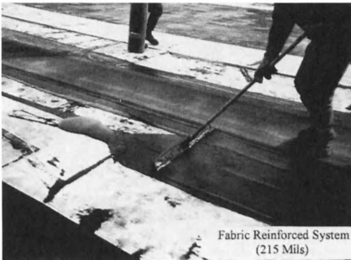
Figure 13-6: Hot-applied membrane application with fabric reinforcement.
