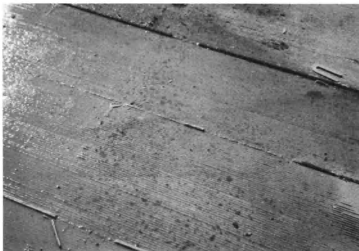
Figure 13-11: Surface preparation is required prior to membrane application.
