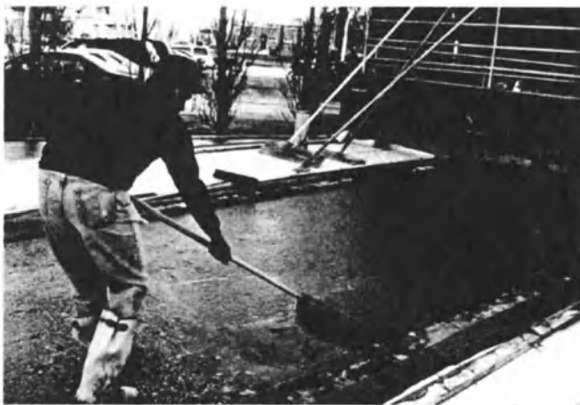
Figure 20-5: Application of bonding grout prior to overlay placement.
