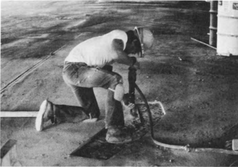
Figure 20-2: Concrete removal by chipping hammer.
