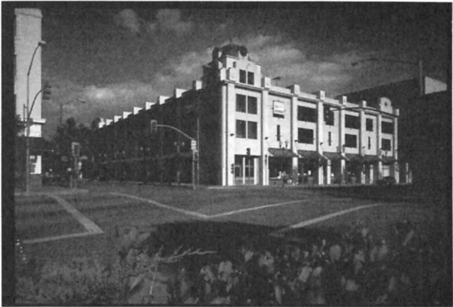
Figure 5-5. Trying to disguise a parking structure as another building type often causes problems maintaining openness. Photo courtesy of Walker Parking Consultants.
