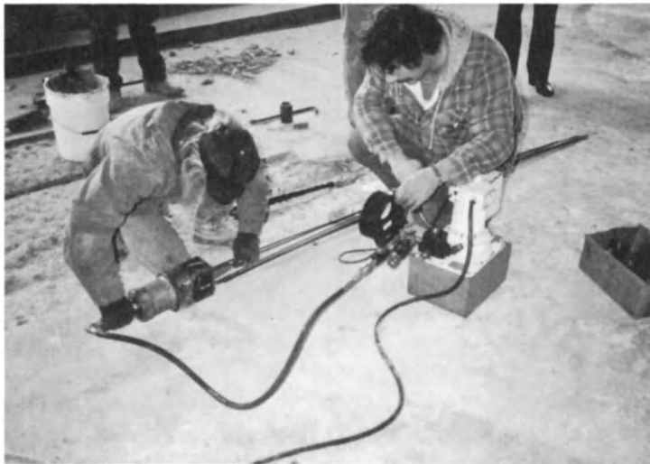
Figure 20-18: (a) Field button heading of wire tendons.
