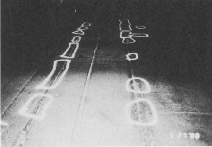
Figure 19-46: Chain drag survey at pour strip with prestressed tendon end anchorages.
