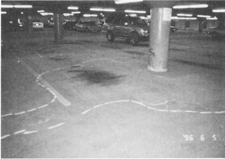
Figure 19-45: Chain drag survey results.
