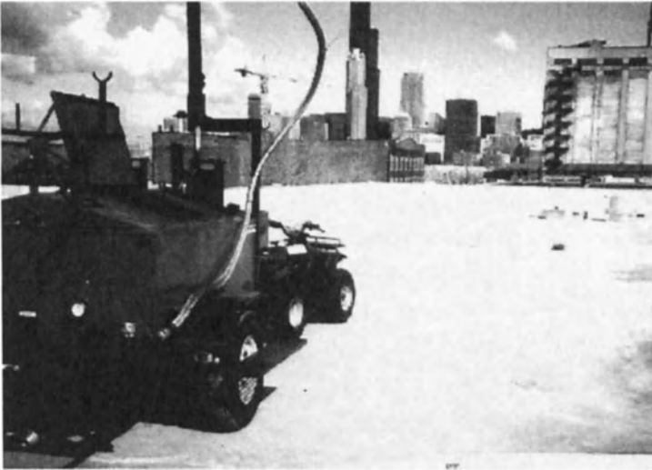
Figure 13-5: Mobile melter for heating the hot-applied membrane materials
