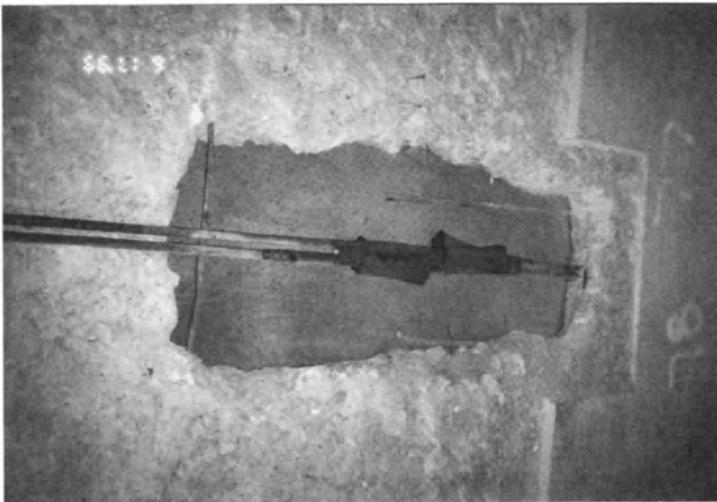
Figure 20-19(b): Tendon splice (strand system).
