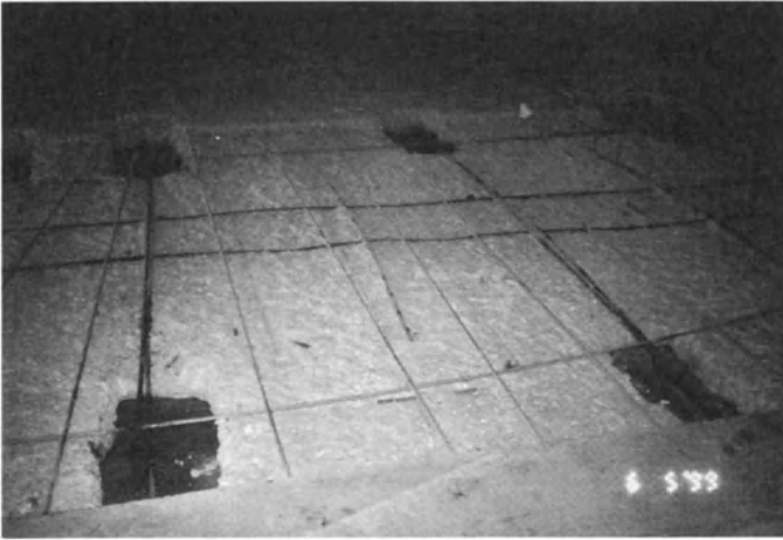
Figure 20-19: (a) Partial tendon replacement over beam.
