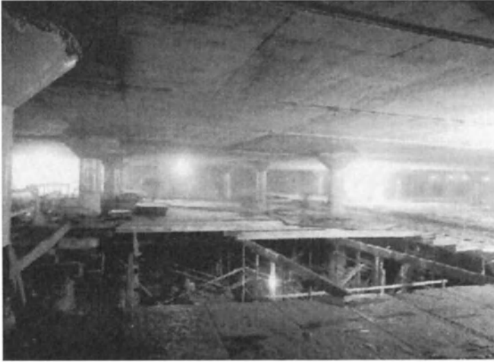
Figure 20-13: Full-depth slab removal (flat slab).
