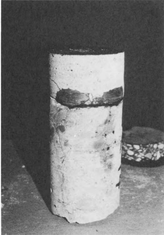
Figure 19-51(c): Core sample over previously patched area with a waterproofing membrane and asphalt wearing surface.
