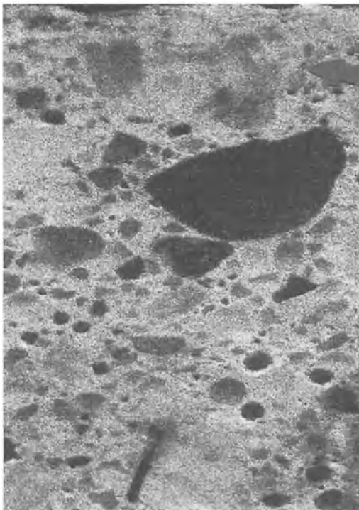
Figure 19-37: Magnified concrete section showing distribution of air entrained bubbles within the concrete. Note lack of air bubbles at top (surface) of the concrete.
