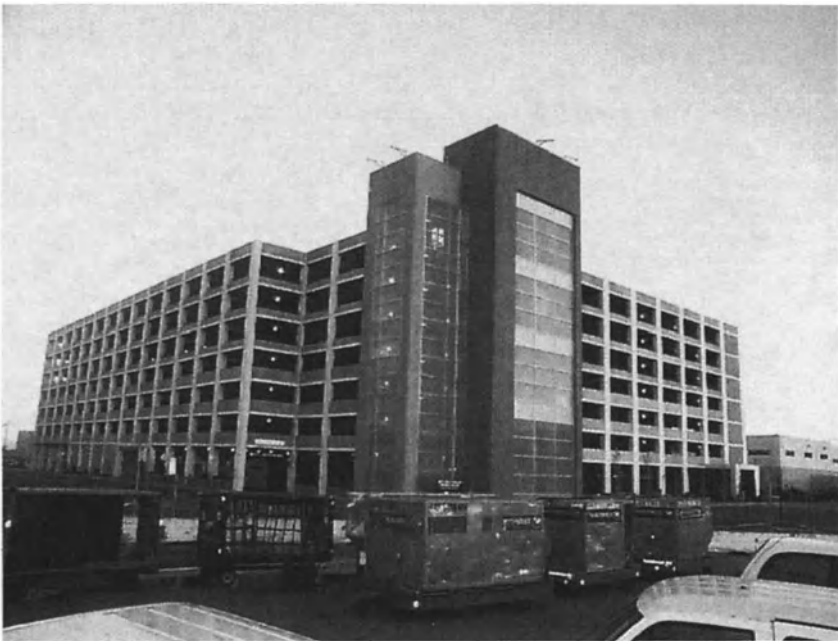
Figure 14.19: San Francisco International Airport employee parking facility, San Francisco, California
