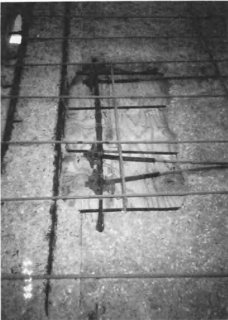
Figure 20-20(b) End anchorage replacement (strand system).
