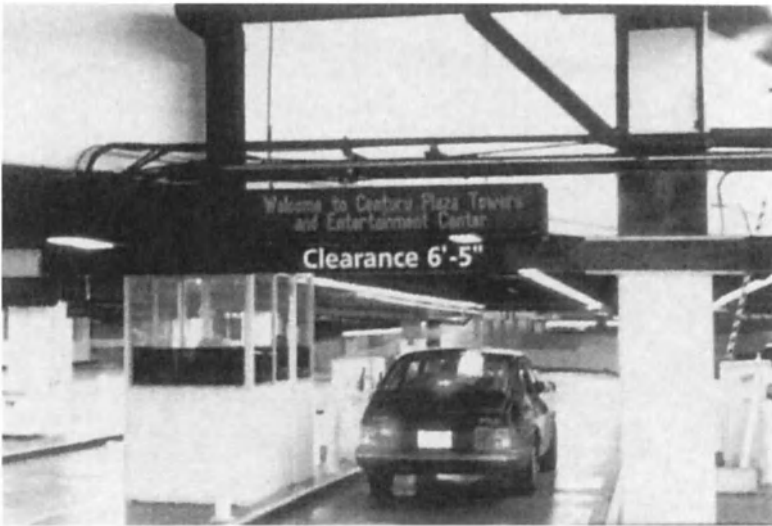
Figure 10-3. Fiber optic signs can compensate for over-illumination behind the sign. Photo courtesy Daktronics, Inc.
