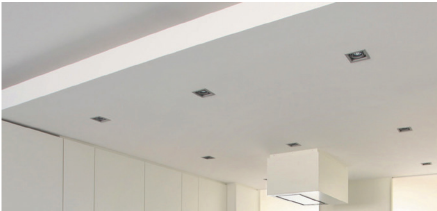
Fig. 3.22 Dropped ceiling by TDP Plasterers Brighton, UK
