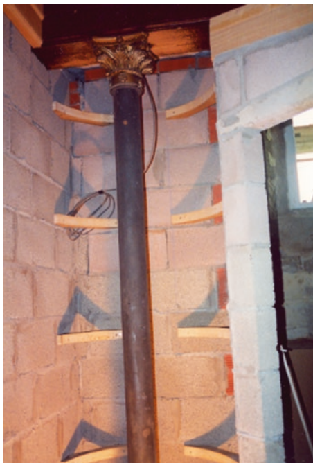
Fig. 4.11 Softwood formers prior to receiving plasterboard. Glendower House. Photograph by author
