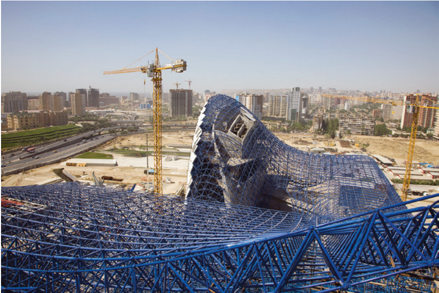
Fig. 3.51 View during construction. Photograph by Luke Hayes, 2010
