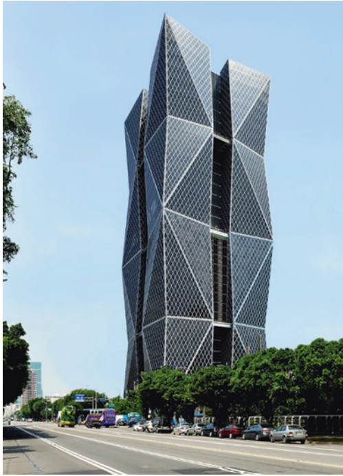
Fig. 1.32 Exterior of building
