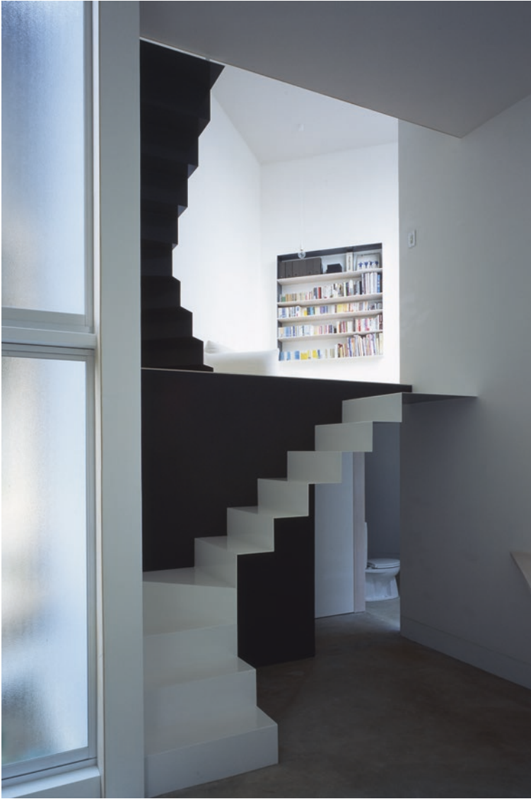
Fig. 4.40 Staircase made of continuous sheet steel in Window House in Kyoto, Japan, designed by Alphaville Architects, 2013
