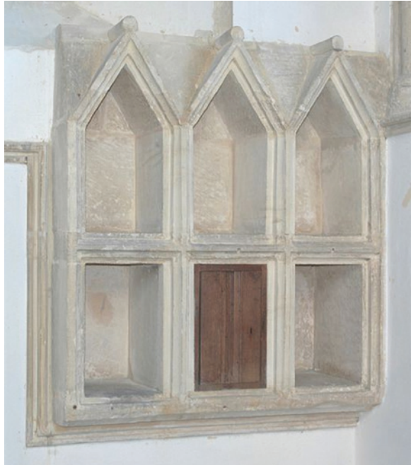
Fig. 3.34 An Aumbry from St Matthew's Church, Langford, Oxfordshire England. Thirteenth century. Owner Motacilla, Wikipedia Commons, 2010
