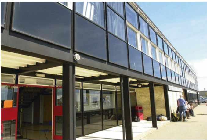
Fig. 4.45 Hunstanton School, Norfolk, UK, 1954. Architects Alison and Peter Smithson. © Archant. By permission of Eastern Daily Press
