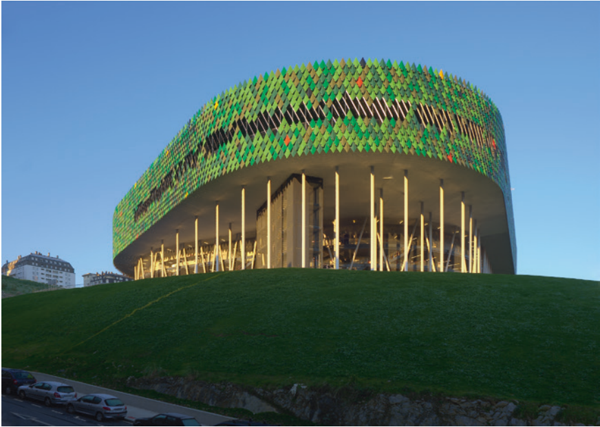
Fig. 3.7 Bilbao Arena and Sports Centre, Spain, 2010. Architects ACXT/Javier Pérez Uribarriy Nicolás Espinosa Barrientos
