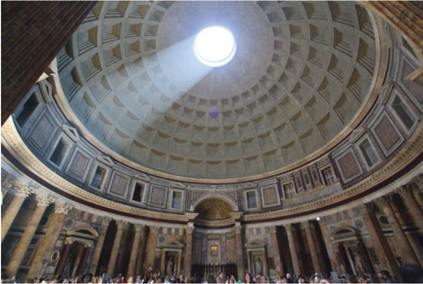
Fig. 7.39 Interior of the Pantheon, Rome, Italy, showing the coffered concrete dome. 126 AD. Photograph by Richijheath of Wikimedia Commons
