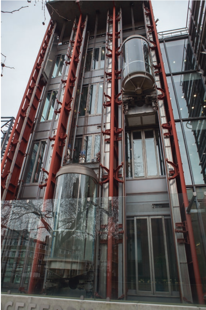
Fig. 2.15 External elevator with transparent car. Channel 4 Office, Victoria, London. By Richard Rogers Partnership, 1994. Photograph by author
