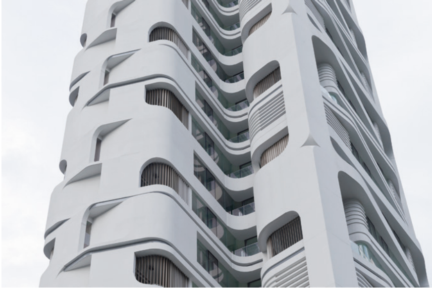
Fig. 1.27 Ardmore Park, Singapore. Architect Ben van Berkel of UNStudio, 2013. Photograph by Iwan Baan. Courtesy © Pontiac Land Group. Exterior view
