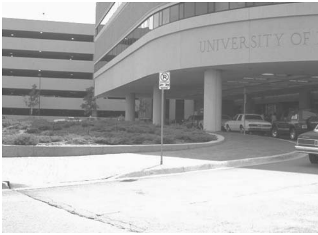
Figure 28.12 This is how the drop-off circle looked during the first few years of the hospital's operation, with no direct entrance to the parking structure. Many years later, in order to provide immediately accessible short-term parking, a direct entrance was created.
