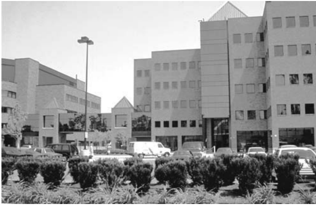
Figure 28.1 The numerous buildings at this medical center are so close together and are designed to look so much alike, that it is almost impossible to tell one from another or to single out a unique destination.
