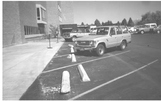
Figure 19.5 Dislocated parking bumpers.
