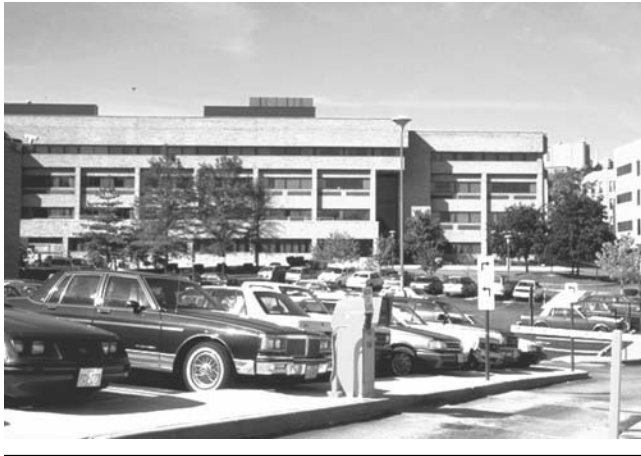
Figure 28.4 One wayfinding-related design obstacle in this children's hospital is the lack of an obvious main entrance, as viewed from the parking area.
