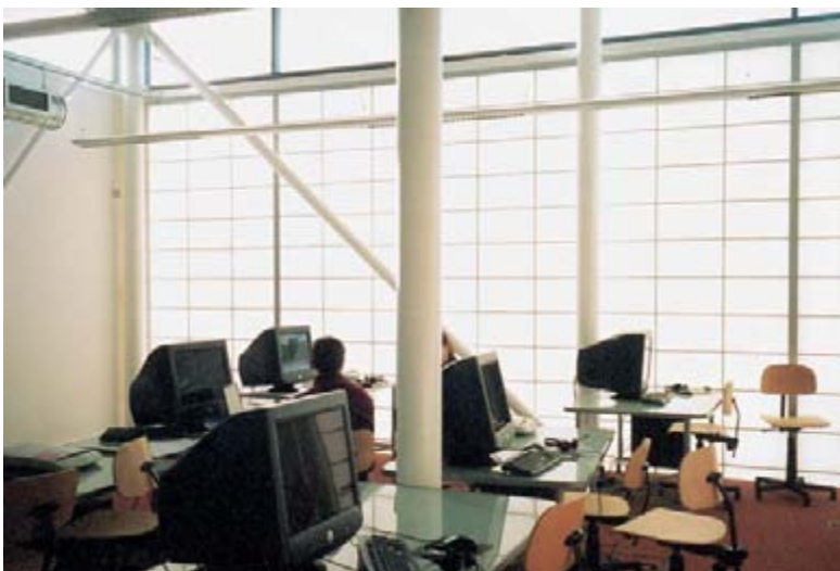
Typical teaching area showing the translucent wall
