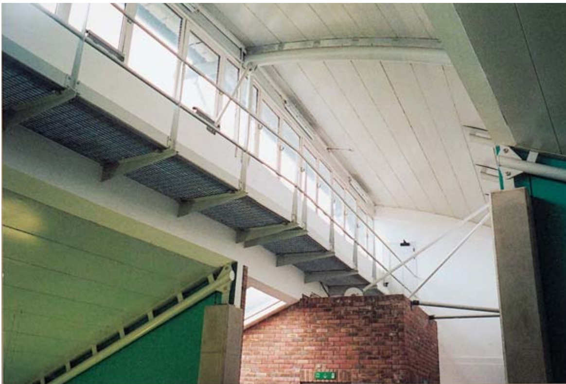
Clerestorey glazing at high level with catwalk for maintenance
