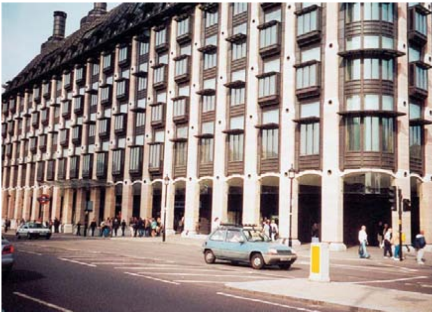
Exterior of the building, to show the colonnading to Bridge Street
