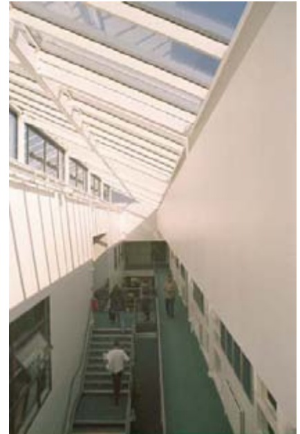
Daylighting to the atrium from roof level
