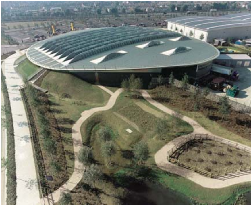
The roof from above
