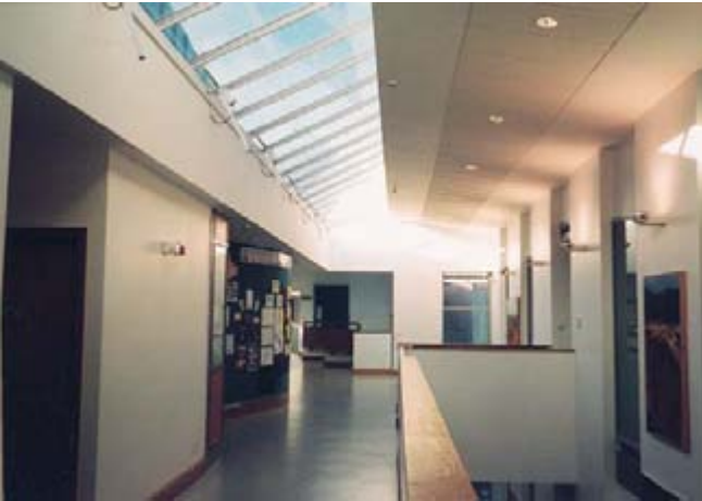
The street at first floor level showing the rooflighting
