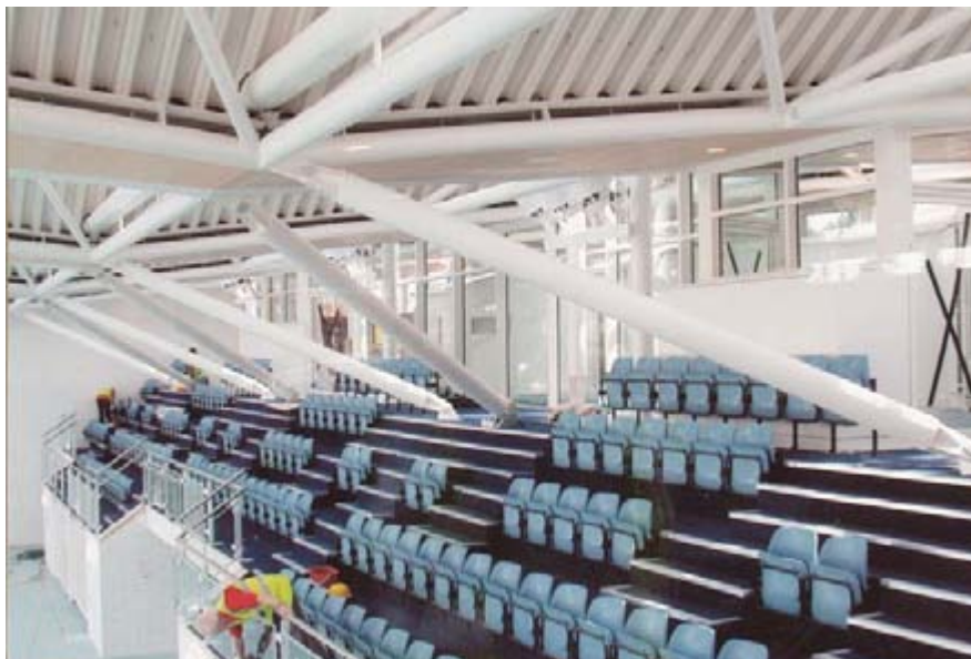
View of roof at seating level
