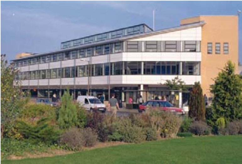
Building exterior, daylight
