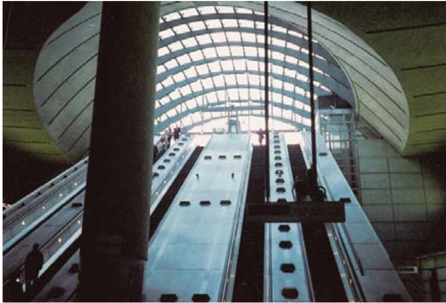
View up escalators to daylit canopy
