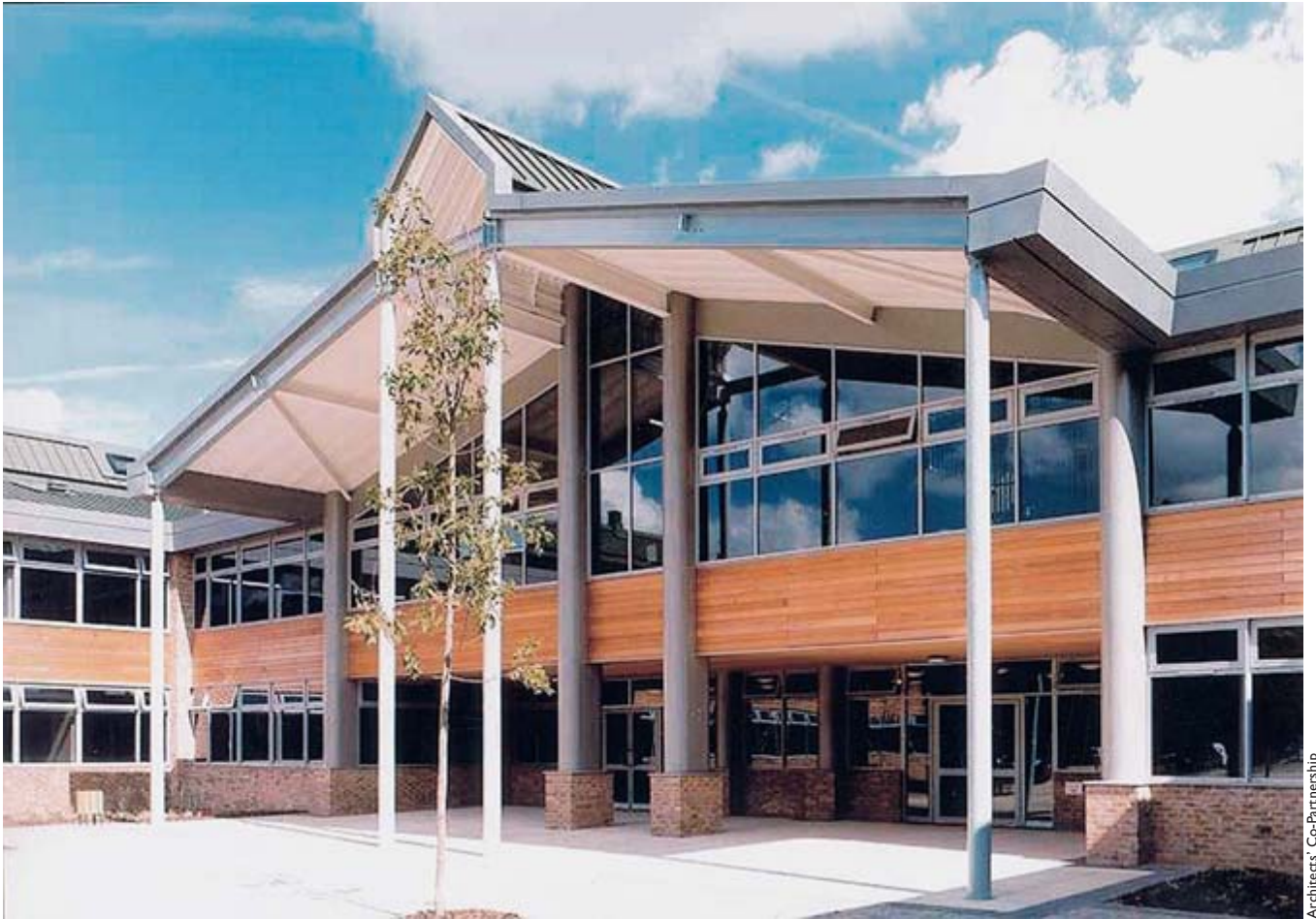
External elevation, main entrance
