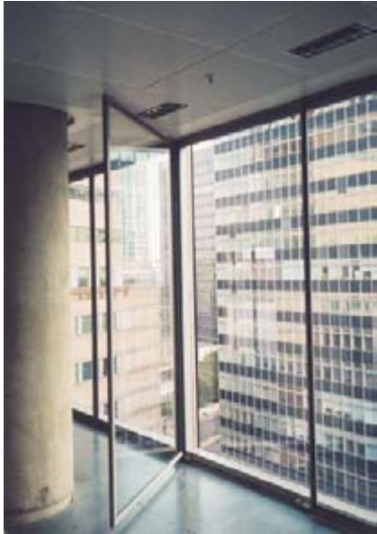
Detail of window with opening leaf
